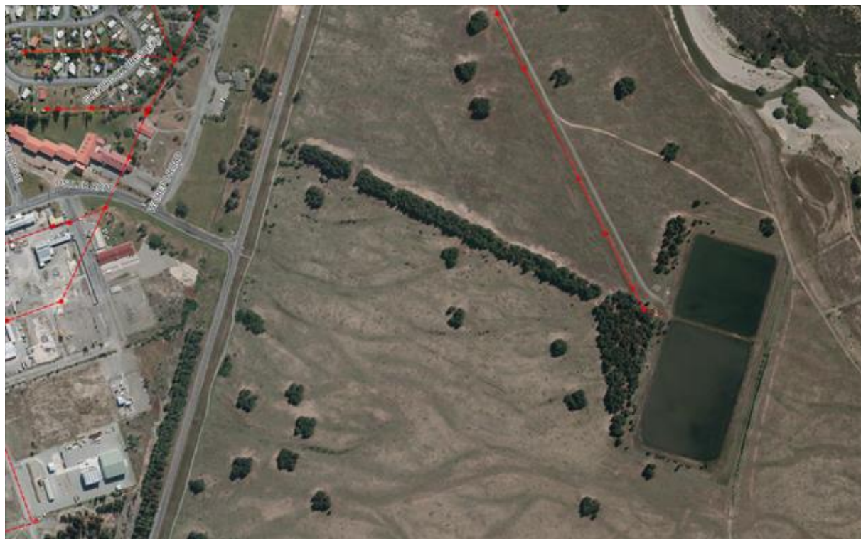
Figure 11-3: Twizel WW Treatment Plant
