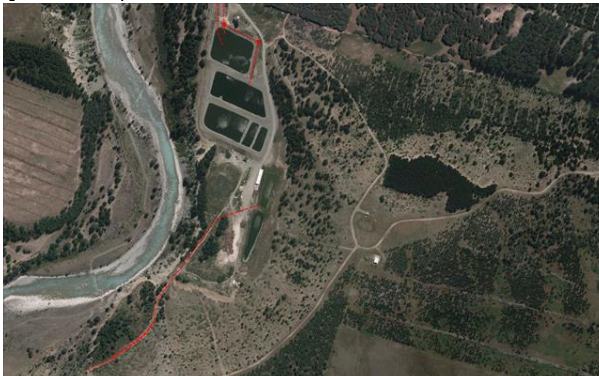
Figure ***Lake Tekapo WW Treatment Plant
