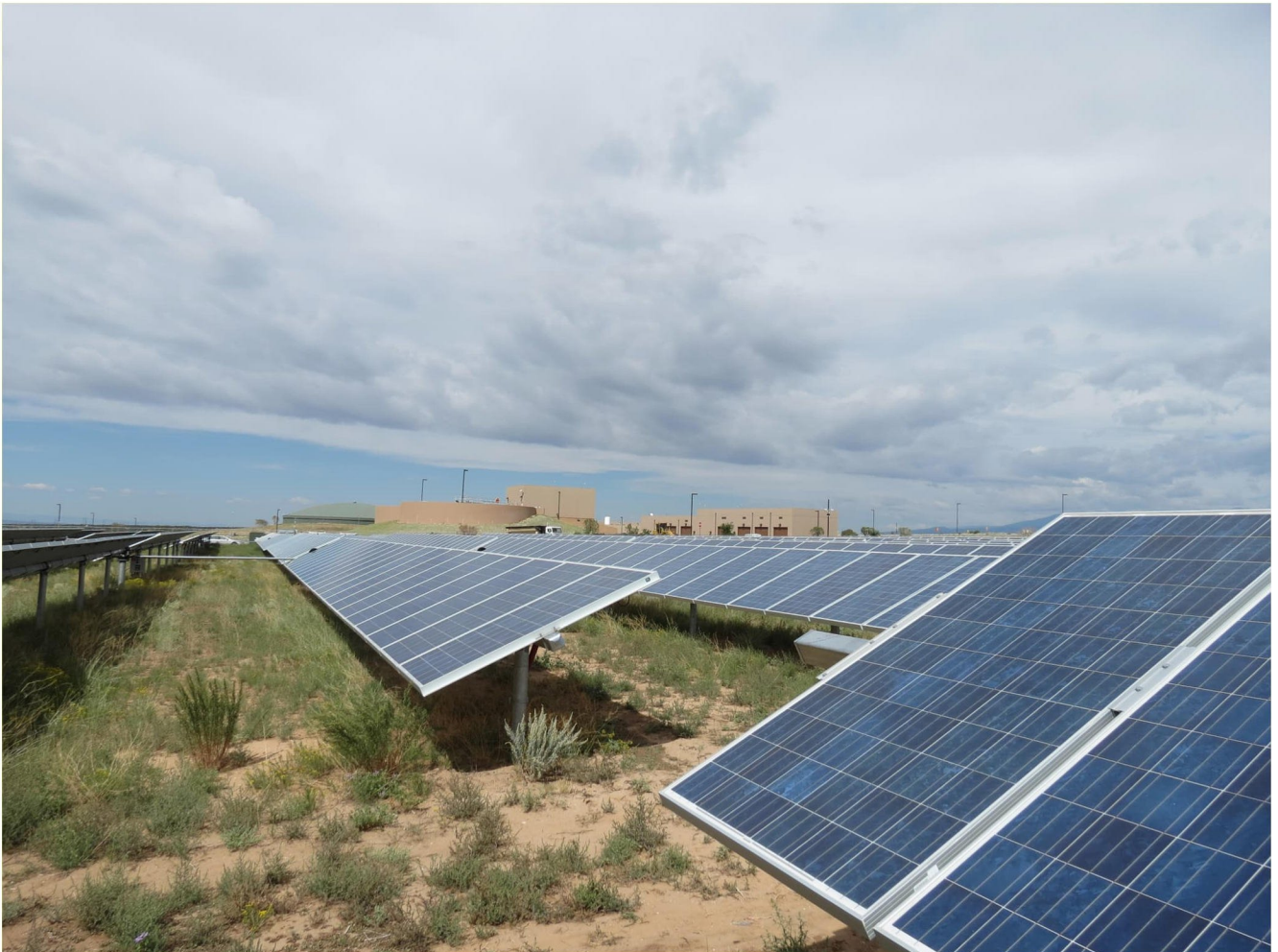
Figure 3. Single axis tracker in 1P format. (Source: FNSF, 2023)
