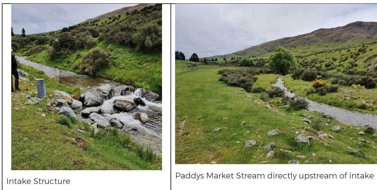
Figure 4-4 Burkes Pass water supply intake photos and view to upstream catchment
