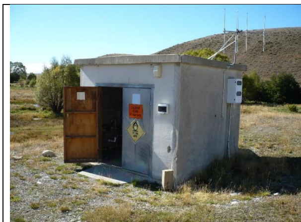
Chlorine treatment building
