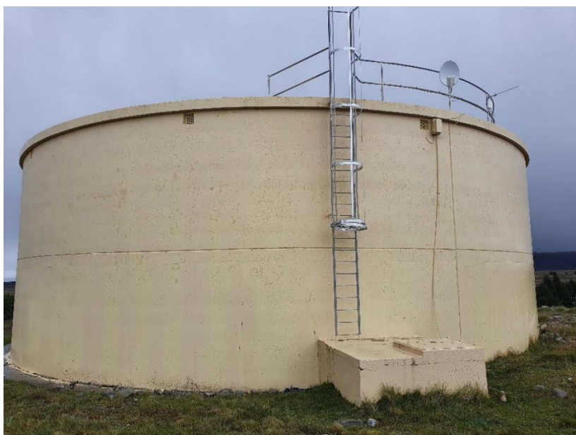
Figure 4-7 Treated water reservoir
