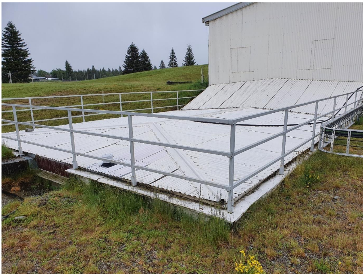
Figure 4-9 Twizel underground treated water reservoir
