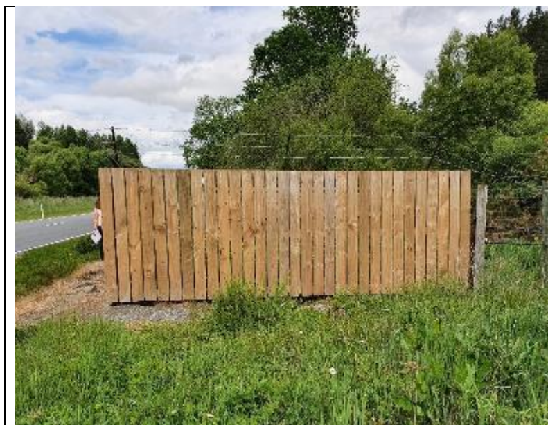
Secure fencing around spring source
