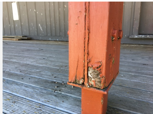
Photo 4. Verandah post base
